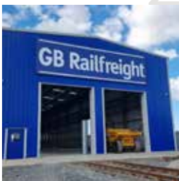
Peterborough Maintenance Hub
